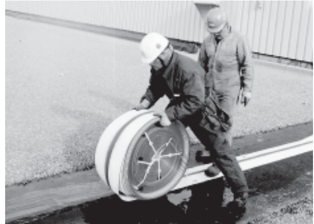
RedLINE 40 being installed in BUR.
