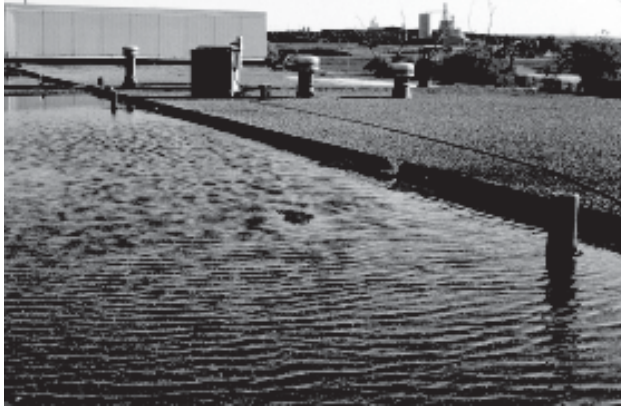
A typical raised expansion joint, preventing water drainage,
