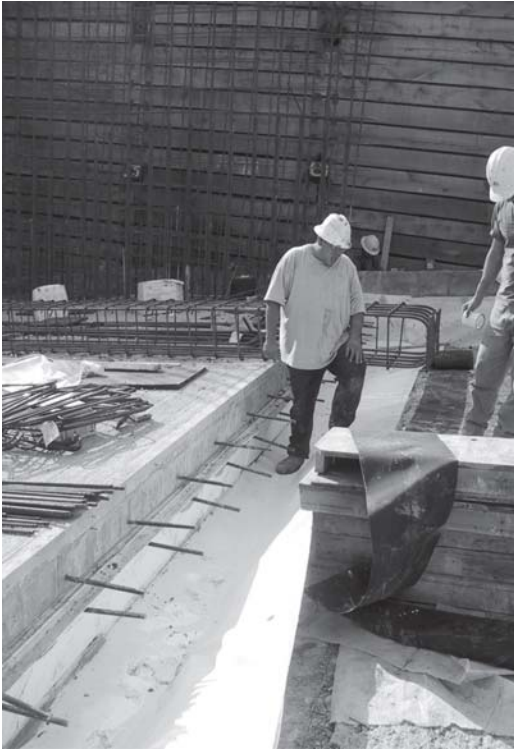
▲ A base ply installation.
