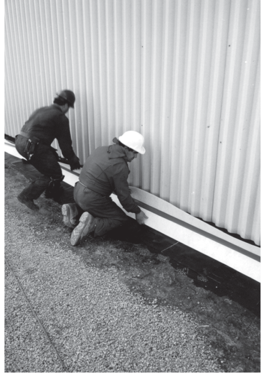
▲ The RedLINE is being fitted in to the joint cavity, the underside of the RedLINE is being laid into hot asphalt.
