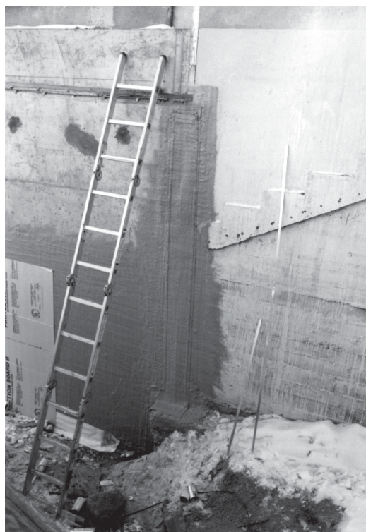
▼ The completed RedLINE installation in a sprayed polyurethane material.
