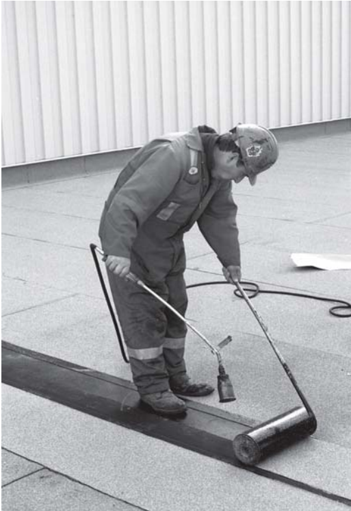
▲ The modified bitumen cap sheet being torched to the FlamLINE.
