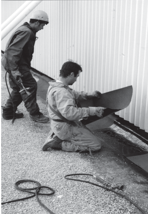
▲ Modified bitumen cap sheet being prepared for torching.
