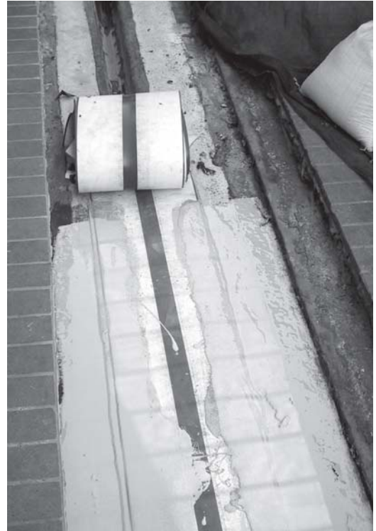
▲ The RedLINE being encapsulated on the top surface in a liquid membrane.
