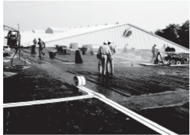
RedLINE 20 being installed in BUR.
