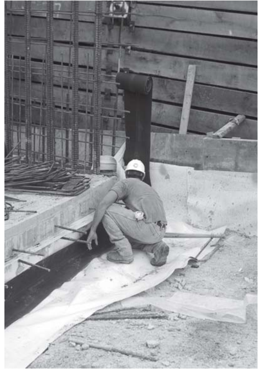
▲ The FlamLINE roll being unrolled and positioned over the joint cavity.
