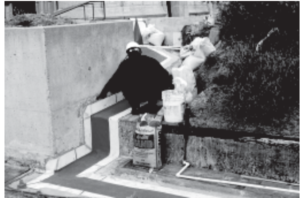
RedLINE 240 being installed.
