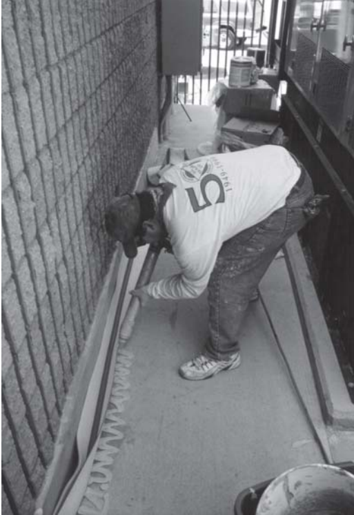
▲ The RedLINE adhered with epoxy to the substrate.
