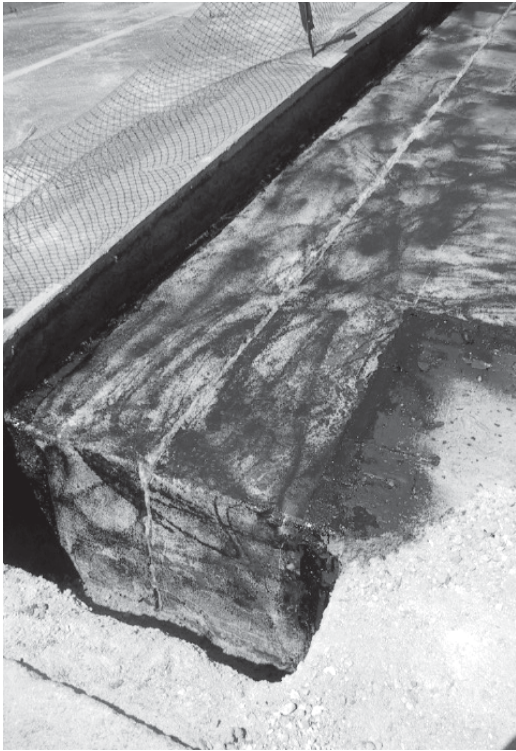
▲ The cleaned expansion joint cavity and primed concrete substrate.
