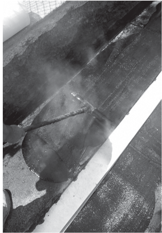
▲ Applying hot asphalt onto the concrete substrate.
