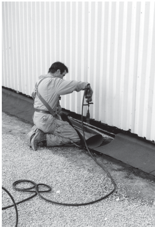
▼ The torched down modified bitumen cap sheet being installed.
