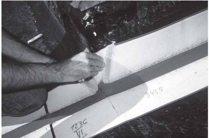
The RedLINE expansion joint custom corner detail at the roof skylight. ▶
