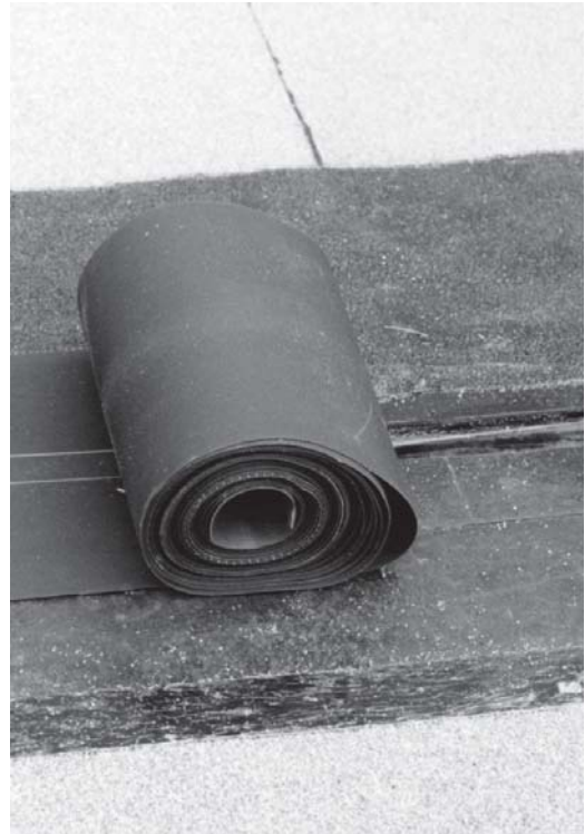
▲ The FlamLINE roll centered over the joint.
