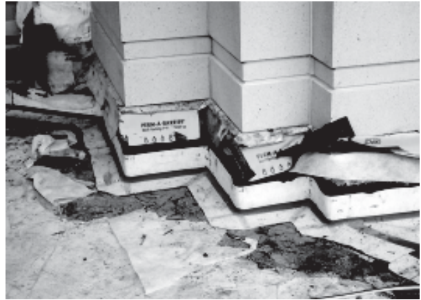
RedLINE 20G installed in Hot Rubberized Asphalt.
