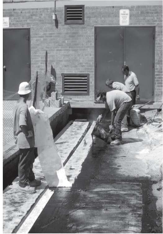
▲ Applying the HRA reinforcing fabric on to the RedLINE as per the hot rubber manufacturer requirements.
