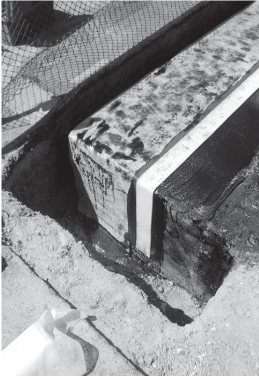
▲ Reinforcing fabric applied to one side of the RedLINE joint (joint termination shown).
