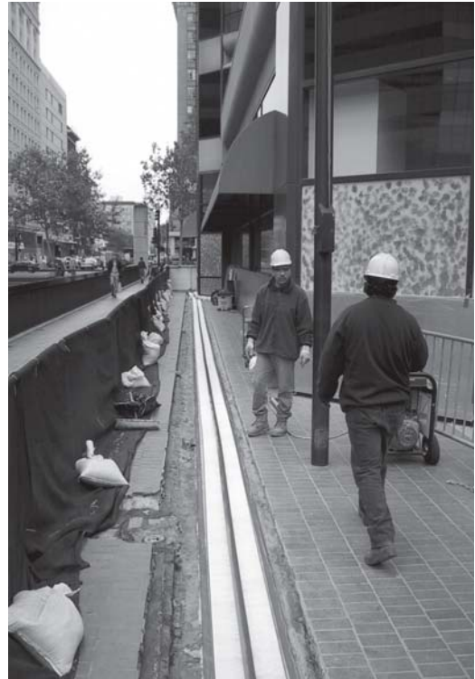
▲ The RedLINE is unrolled to check for fit.
