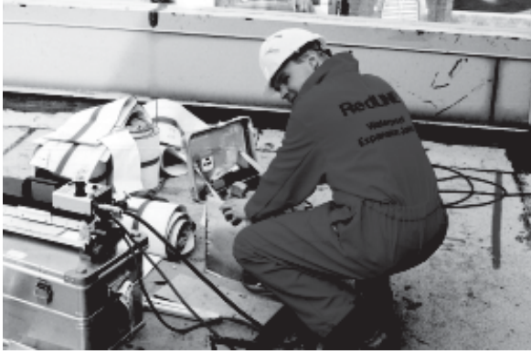
SITURA material being vulcanized on site.
