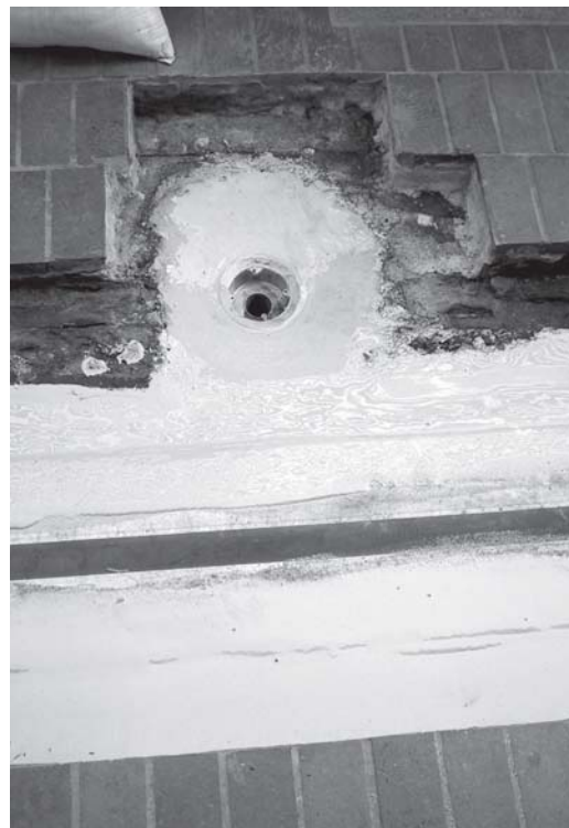
▲ A drain detail next to the RedLINE, note the liquid membrane continuity.
