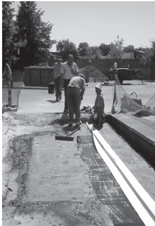
▼ The RedLINE is being rolled out into the hot asphalt.
