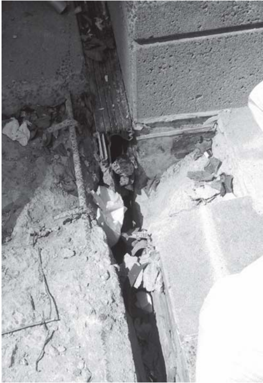
▲ The expansion joint cavity exposed at a detail, prior to membrane application.
