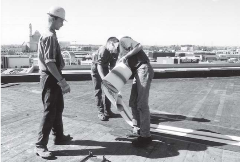
The RedLINE expansion joint custom corner detail at the roof skylight. ▶
