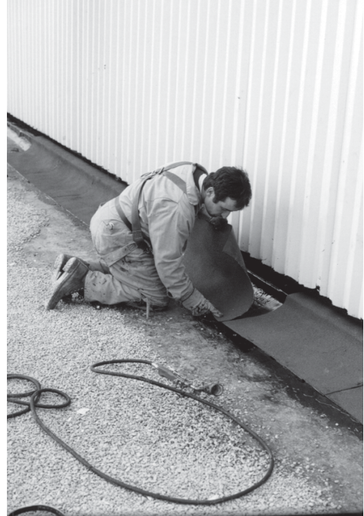
▲ Modified bitumen cap sheet is torched down to the asphalt primed RedLINE fleece.
