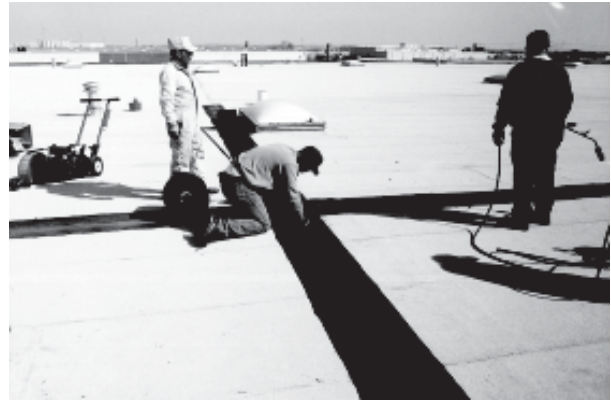
FlamLINE 100 installed in a torched system.
