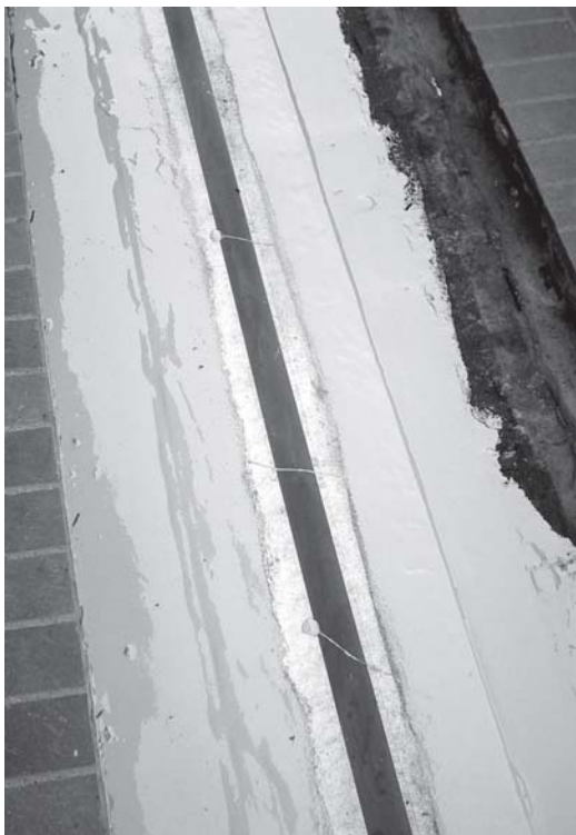
▲ A close up of the RedLINE expansion joint encapsulated in liquid membrane.
