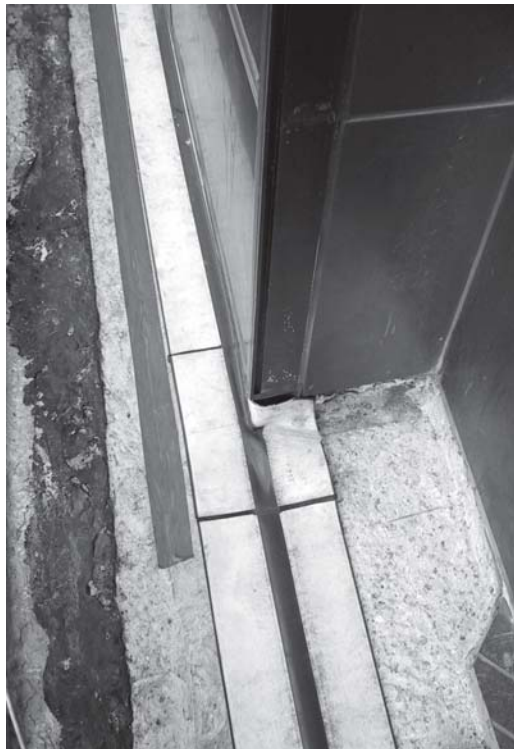
▼ RedLINE laid out at a detail on site prior to encapsulation.
