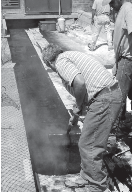
▲ Applying the second coat of hot rubberized asphalt over the reinforcing fabric.
