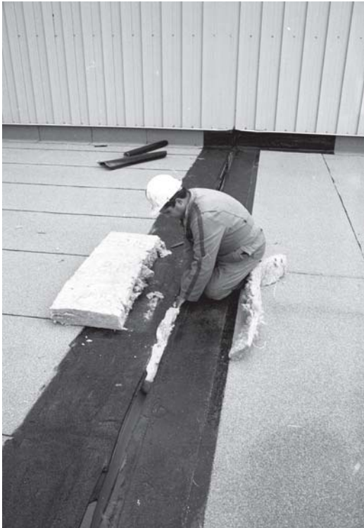
▲ The joint cavity is open and batt insulation is placed in it.
