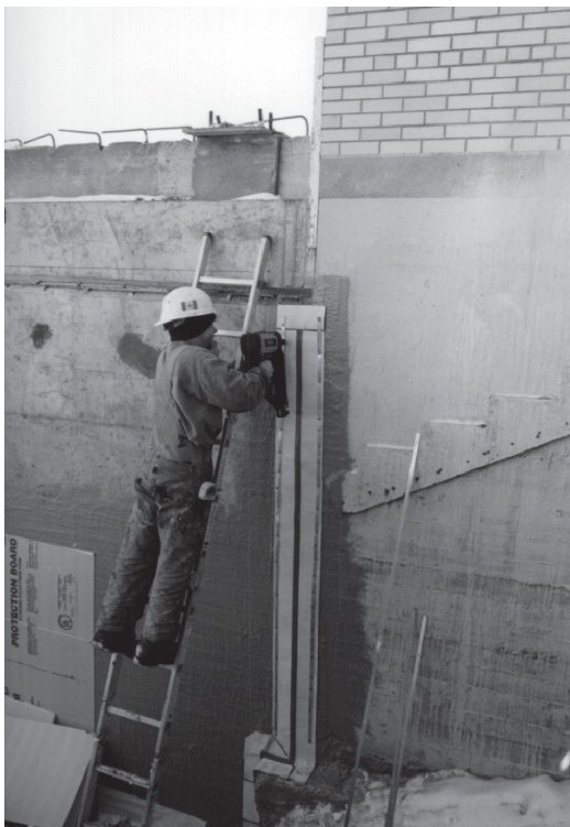
▲ The RedLINE is secured to the concrete substrate with termination bars all the throughout its height.
