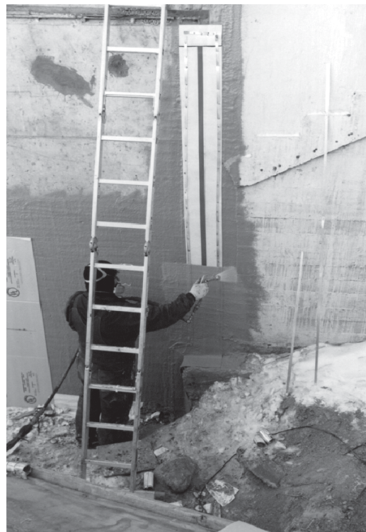
▲ The RedLINE being covered with the polyurethane.
