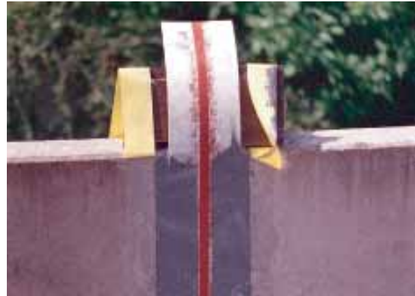
RedLINE 06 being installed in epoxy.
