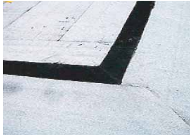
FlamLINE 240 installed in a torched system.
