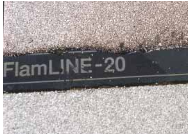
FlamLINE 20 installed in a torched system.
